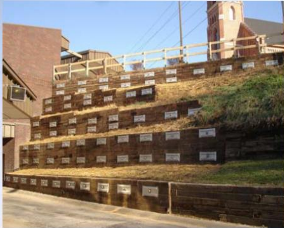
Retaining wall - after
