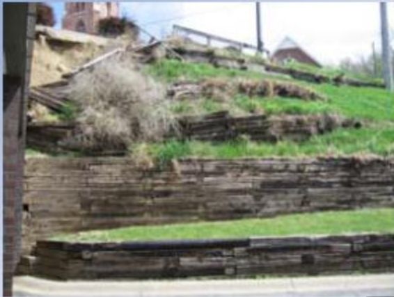
Retaining wall - before
