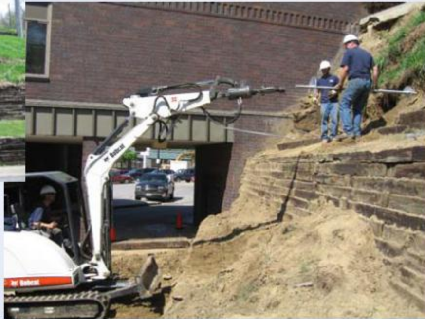
Helical tiebacks on retaining wall
