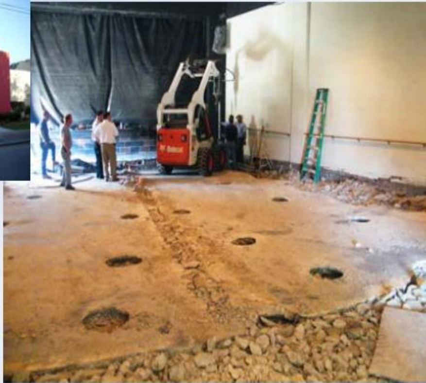
Helical pile installation within auditorium of community theatre
